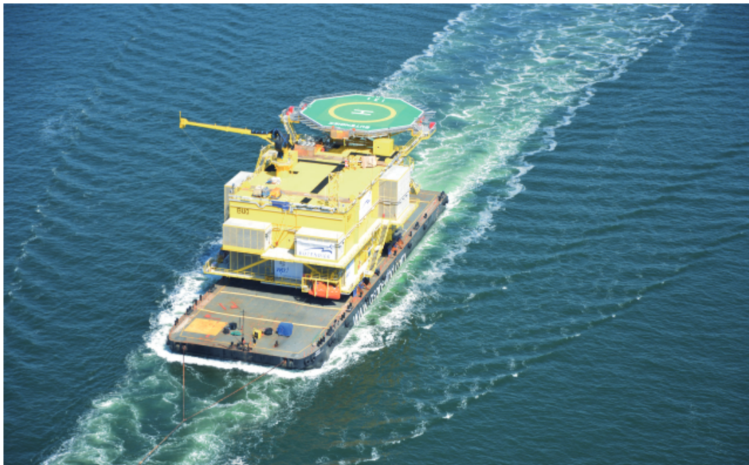
Figure 3.1.6.1: Transporting a transformer substation for a wind farm in the North Sea. | Source: Dr. Born - Dr. Ermel GmbH.
