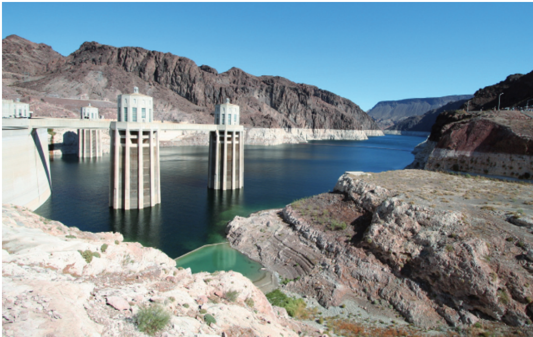
Figure 3.1.8.2: Reservoir with intakes of a hydroelectric power plant. | Source: Fotolia.
